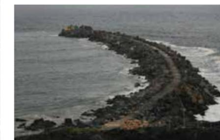
BMT WBM was engaged to assist with the preparation of a Review of Environmental Factors for undertaking remedial works to the eastern breakwater. The proposal included casting and storage of concrete "Hanbar" armour units, supply and placement of quarried rock to upgrade of an accessway along the crest of the breakwater and rearmouring of the breakwater trunk by placement of Hanbar armour units along both sides of the breakwater to protect the core and integrity of the structure.
